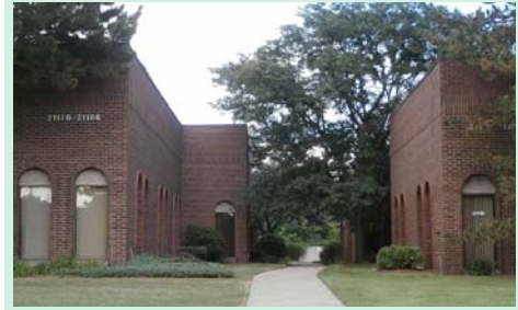
Bridge Commerce Center, Southfield
